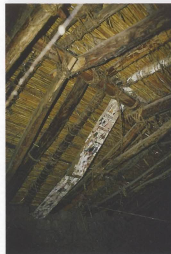
Photo 1. Alza techos (roof-lifters) under a corrugated tin roof. Photo: Olga González.
